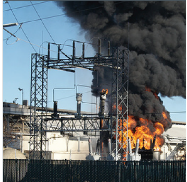
Transformer explosion caused by excess moisture in the transformer's oil.
